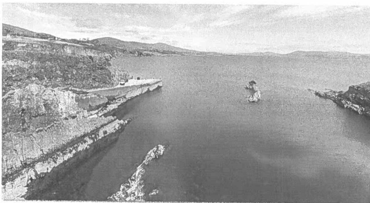
The distance between the turning bollard and the pier
